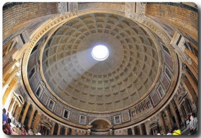
Figure 4: Vault with coffered ceiling and oculus.
