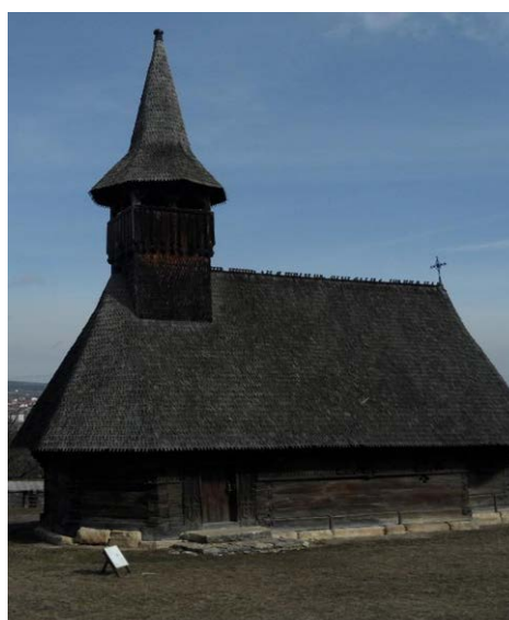
Fig. 4: The wooden Chiraleș Church
