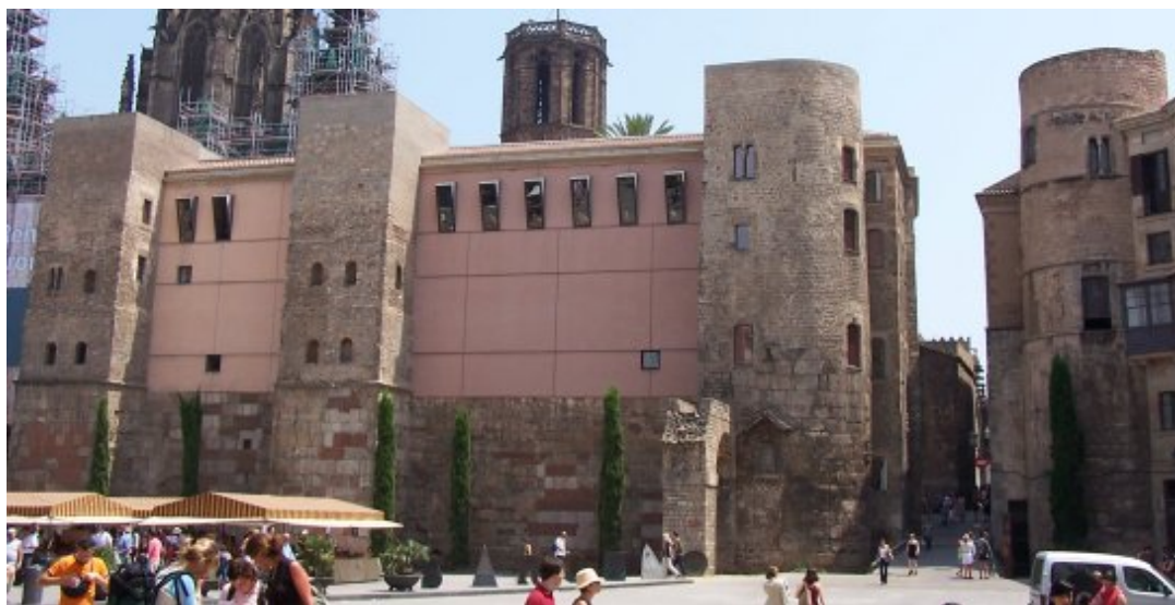
Fig. 18: Now one of the three arcades that the Porta Praetoria had is appreciated, and the two towers of circular plant that defended the sides. It is possible to see some rest of the aqueduct, which arrived to Barcino.
