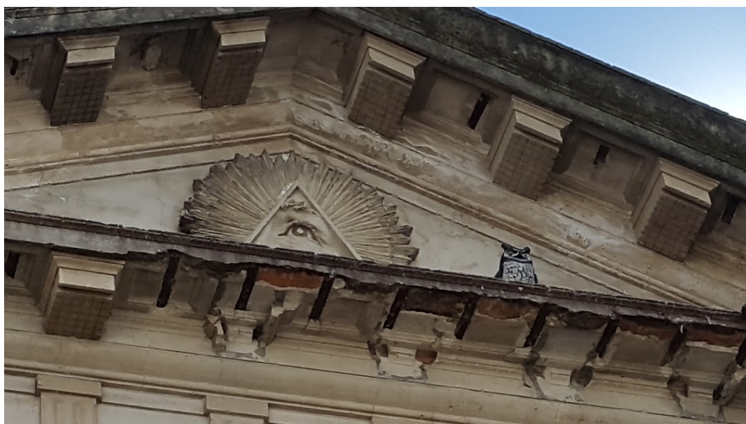
Fig 1. Masonic Temple in Concordia: Entrance detail.
